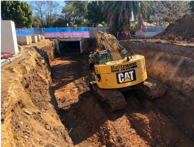
Channel excavation
