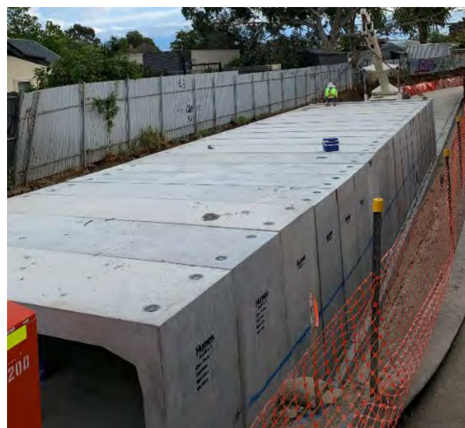
Culvert installation
