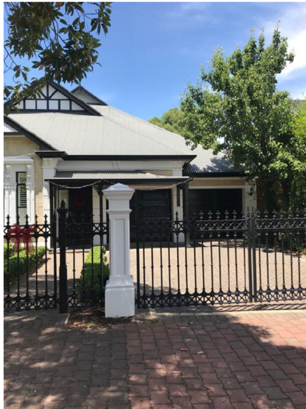
21 Invergowrie Avenue, Highgate – note the dominant roof form over the garage, notwithstanding the verandah.
