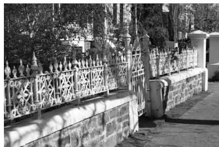
Masonry & cast iron palisade inserts
