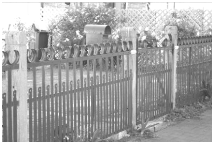
Timber posts with steel strap panels
