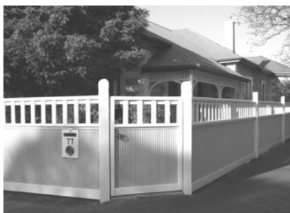
Corrugated mini orb with timber framing
