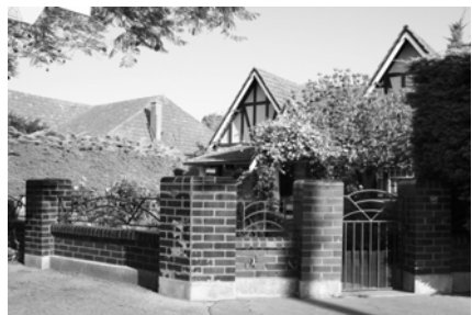
Brick & masonry base with wrought steel inserts
