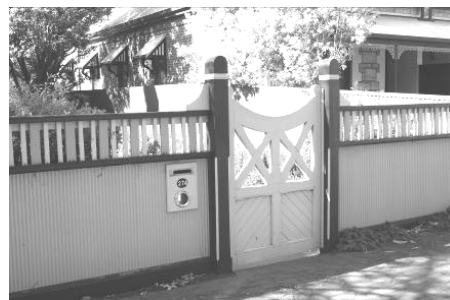
Corrugated mini orb with timber framing
