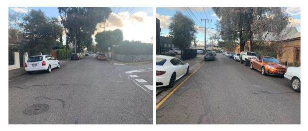
**Stamford Street intersection**: the current intersection is not designed to cater for heavy/large vehicles and or increased traffic flows due to its proximity to Greenhill Road and T-junction arrangement with Stamford Avenue. As mentioned, the current directional split of traffic is 70 per cent northbound, and hence the new development under its current configuration would likely double (if not triple) the current vehicle movements traversing this intersection.
