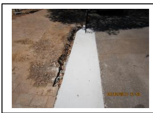
CUTTING STRAIGHT EDGE TO BITUMEN ROADS FOR CONCRETE WORKS
