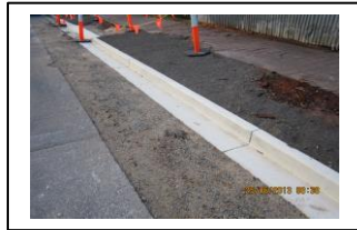
INSTALL NEW DRIVEWAY CROSSOVER & KERBING
