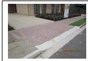
INSTALL NEW DRIVEWAY CROSSOVER & KERBING
