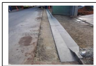
CUTTING STRAIGHT EDGE TO BITUMEN ROADS FOR CONCRETE WORKS
