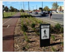
Photo 28: Shared Path as well as on-road lanes for faster cyclists, Hindmarsh SA.
