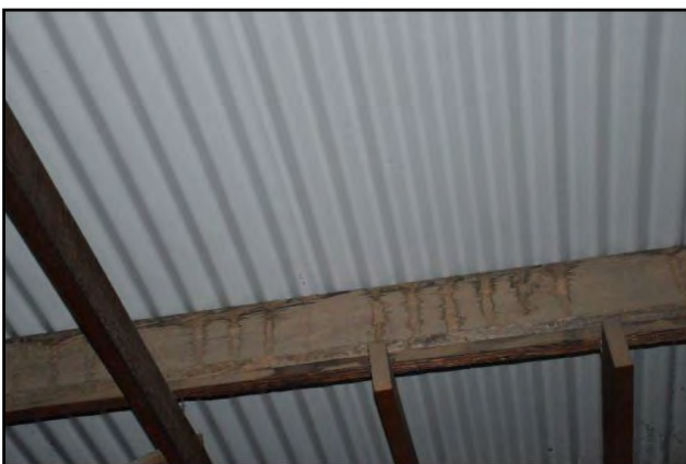
Figure 31 – Moisture ingress to roof purlins
