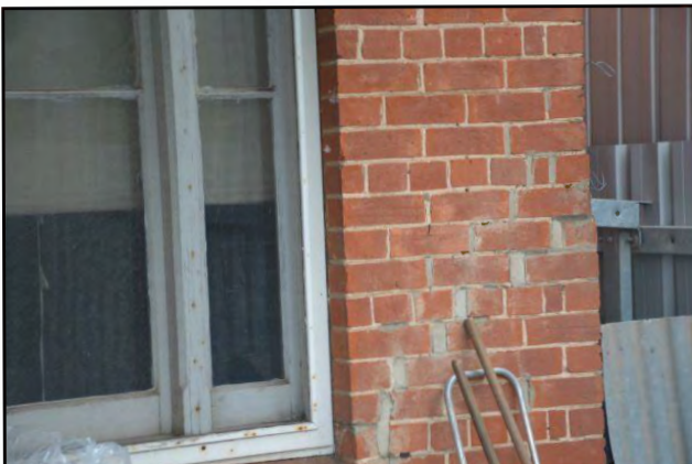
Figure 7 – External wall cracking damage (repaired) Category '4'
