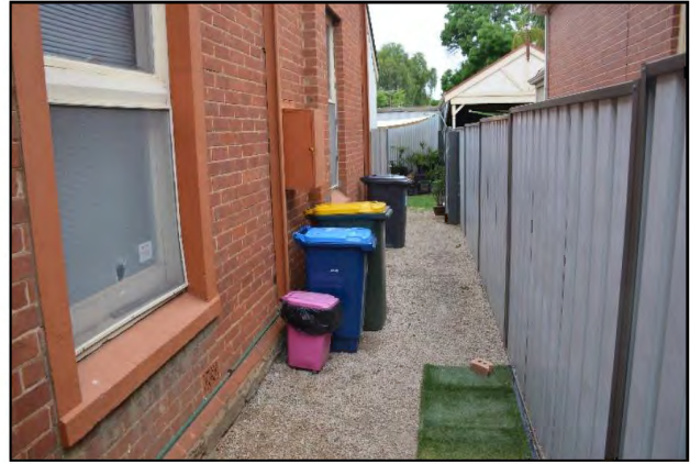
Figure 15 – Absence of perimeter pavement
