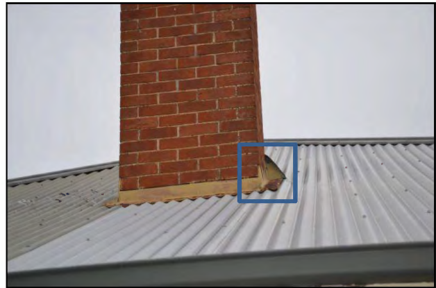
Figure 25 – Corroded roof flashing and inadequate fixations
