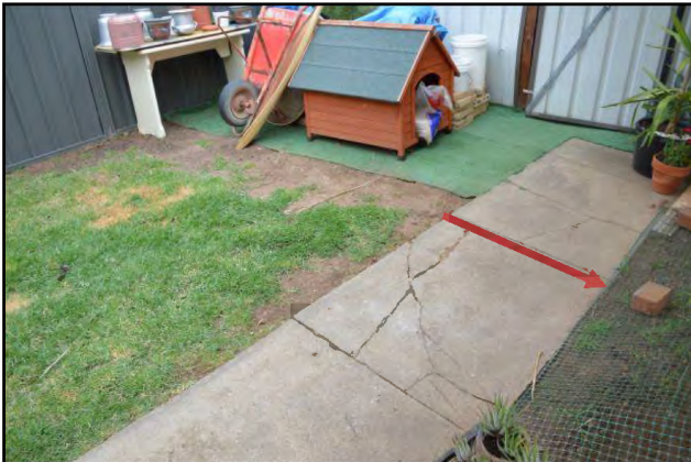
Figure 16 – Settling & damaged concrete path
