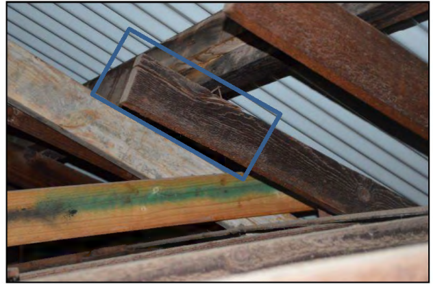
Figure 29 – Deteriorated roof timber members- early sign of splitting
