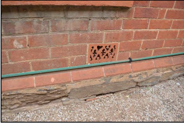
Figure 14 – Absence of perimeter pavement
