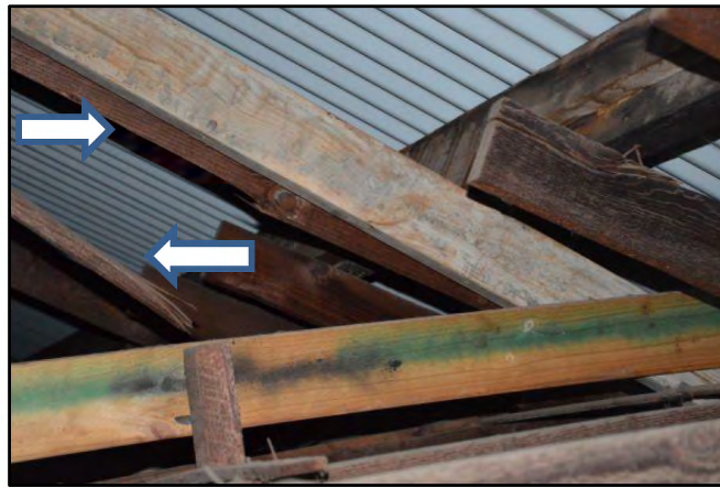
Figure 30 – Split apart roof timber rafter
