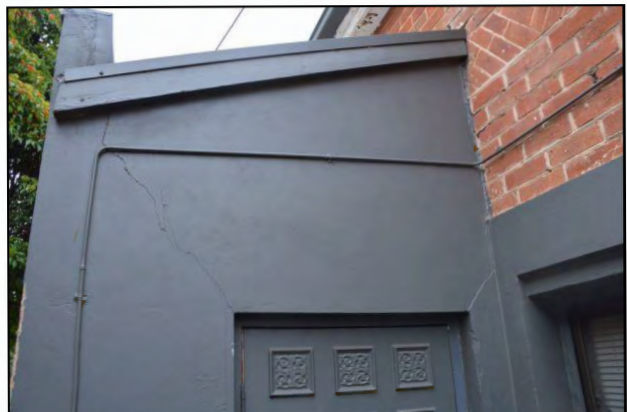
Figure 8 – External wall cracking damage
