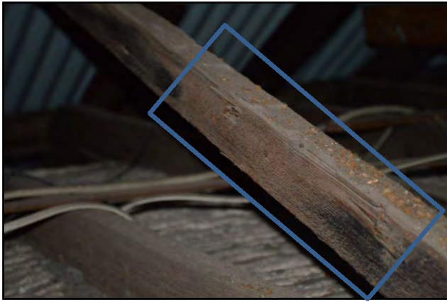
Figure 28 – Deteriorated roof timber rafter
