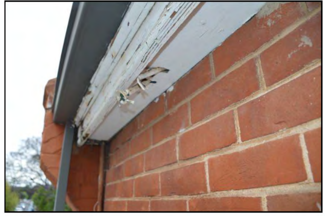
Figure 19 – Deteriorated timber fascia supporting roof gutter
