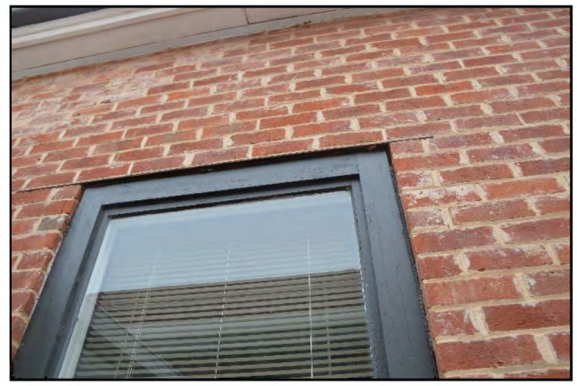
Figure 12 – Corroded window structural steel lintel
