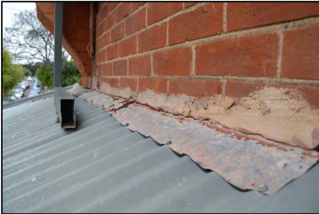
Figure 24 – Corroded roof flashing and inadequate fixation
