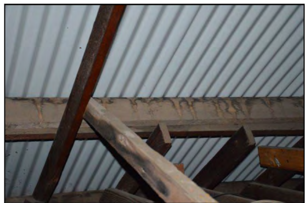
Figure 32 – Moisture ingress to roof purlins
