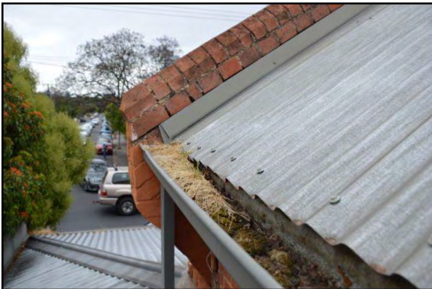
Figure 20 – Blocked roof gutter
