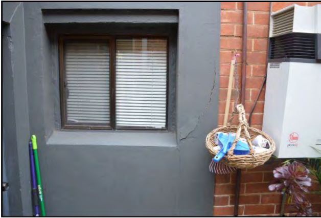
Figure 9 – External wall cracking damage
