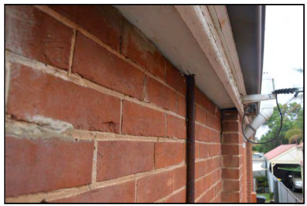
Figure 23 – Significantly corroded service pipes
