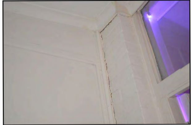
Figure 5 – Typical cracking damage to internal walls
