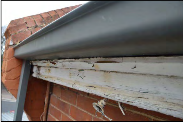
Figure 18 – Deteriorated timber fascia supporting roof gutter
