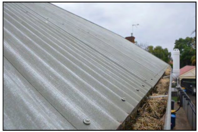
Figure 21 – Blocked roof gutter
