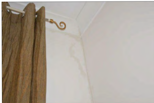
Figure 6 – Signs of previous paint repair
