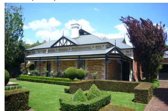
Photo 10 : Return verandah villa at No19 ( c 1913/14 )
