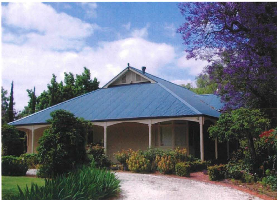
7 Thornber Street (Photo: 31 November 2010).
