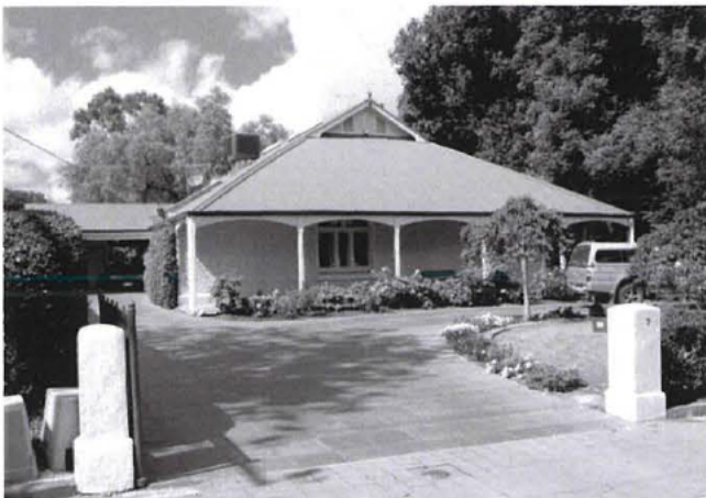
7 Thornber Street. Built probably about 1913 or 1914 (Photo: 2012).
