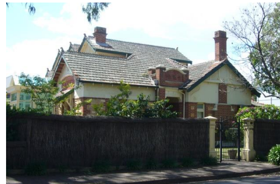
Photo 18 : Federation/Arts & Crafts villa at No 14 Thornber St / corner of George St ( c 1912/13 )
