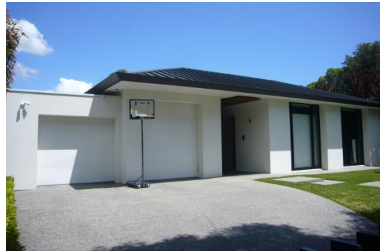
Photo 6 : The adjacent dwelling at No 5 Thornber St
