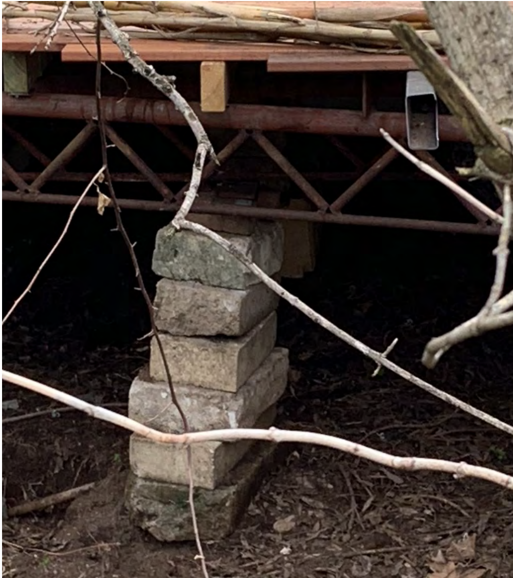
186 Deck Support - untreated Pine & salvaged materials
