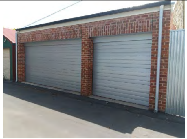
Existing Red Brick Garage in Rose Lane
