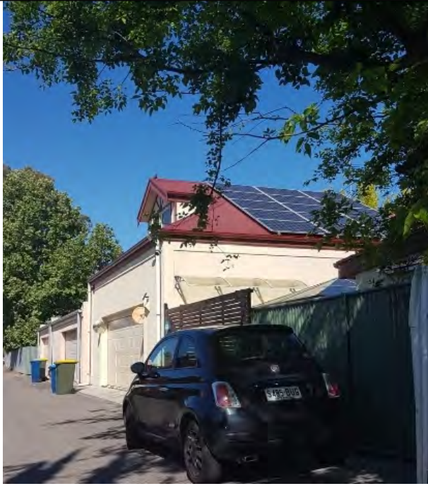
Existing Loft Space Above Garage in Davenport Lane
