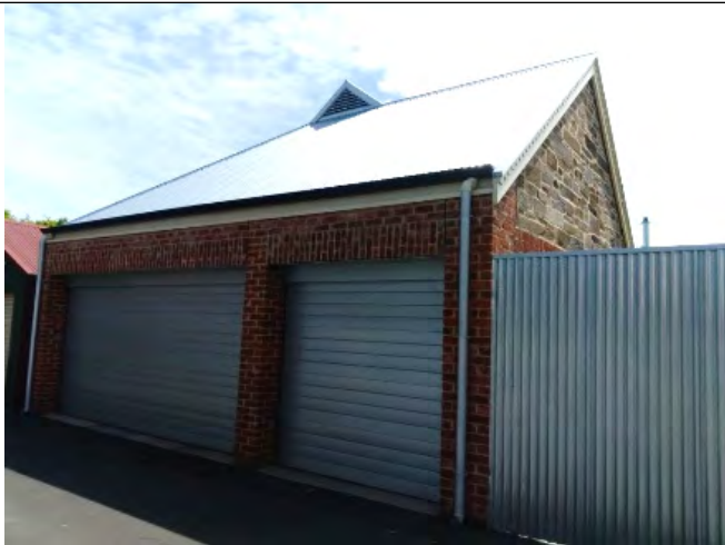
Existing Red Brick Garage with Stone Gable in Rose Lane
