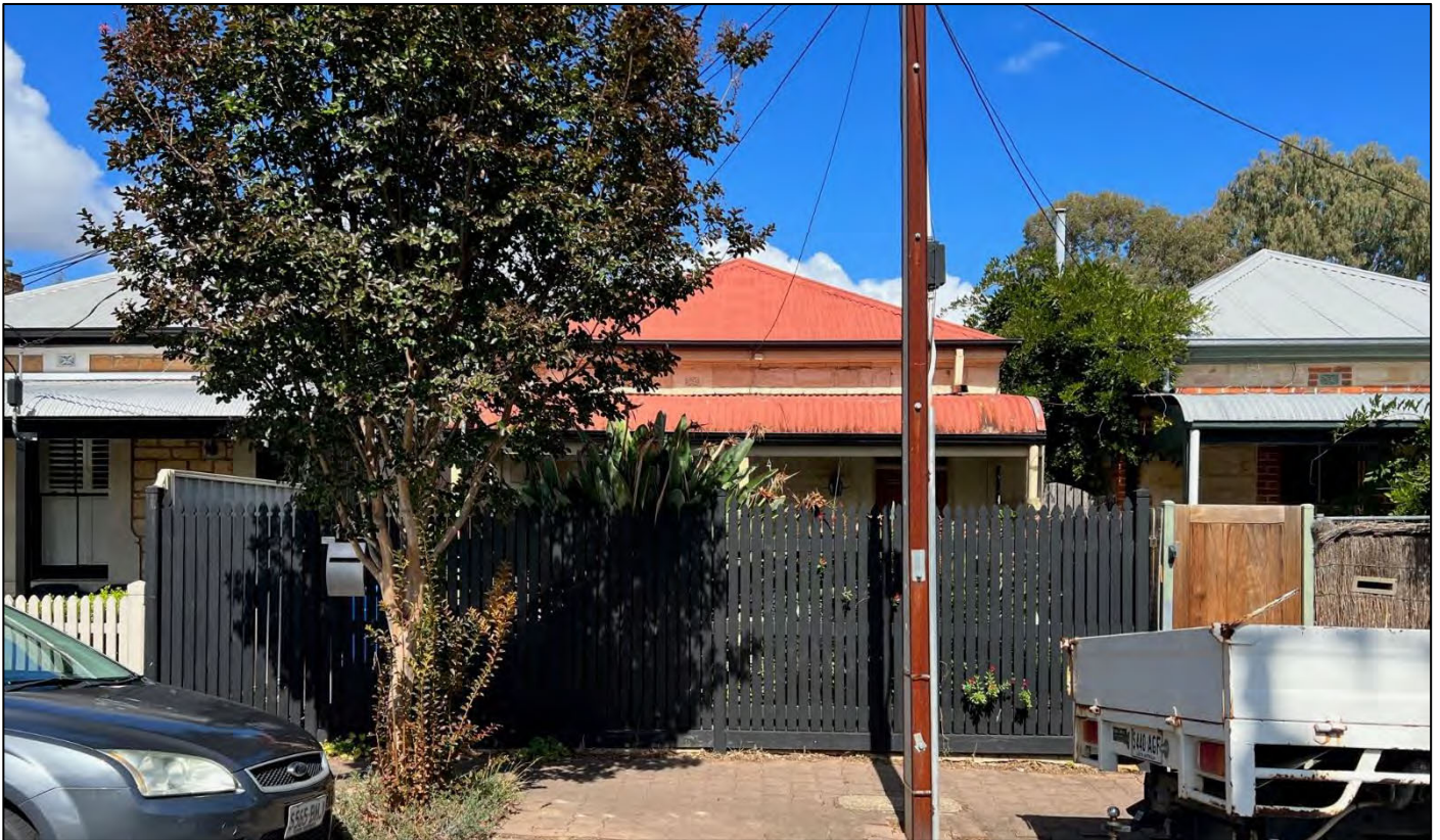
Figure 3: View of the neighbouring property to the west (115 Leicester St) taken from Leicester St looking south
