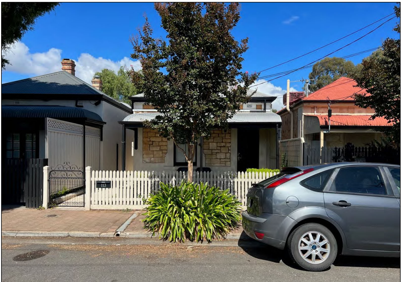
Figure 1: View of the subject land as taken from Leicester St looking south
