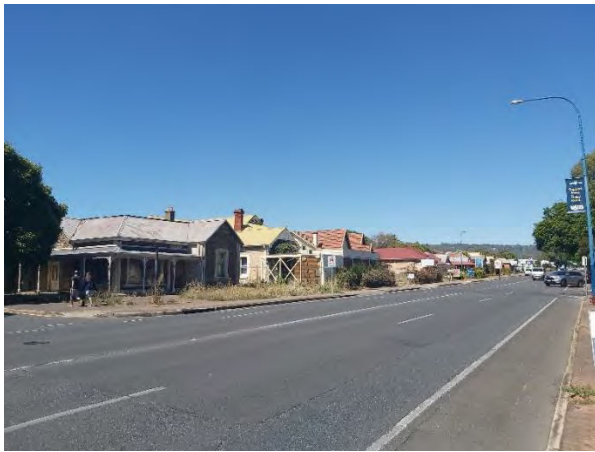
Figure 1: The subject site looking south east.
