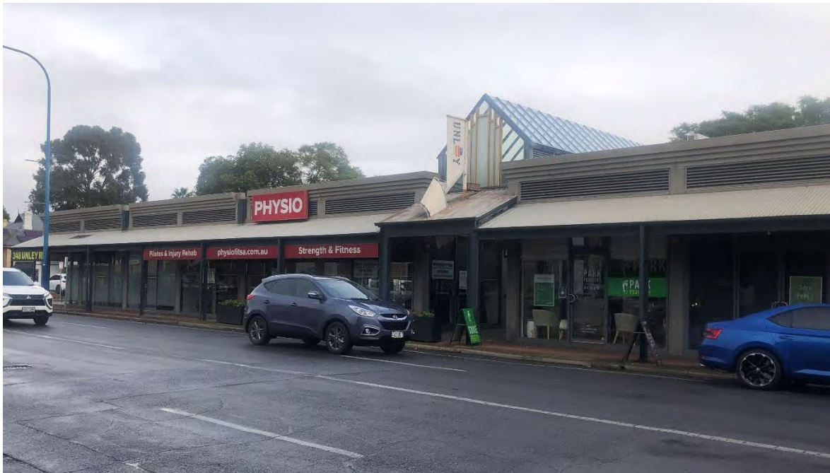
Figure 3.10 Group of shops at 346-354 Unley Road single across the road
