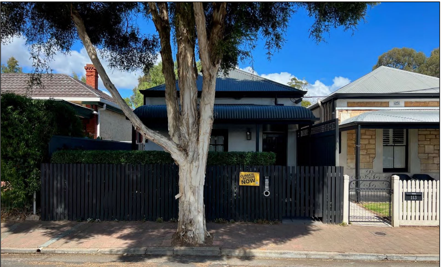
Figure 4: View of the neighbouring property to the east (111 Leicester St) taken from Leicester St looking south
