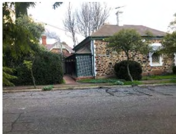
View of existing dwelling at 1A Gladstone Street facing east on Gladstone Street
