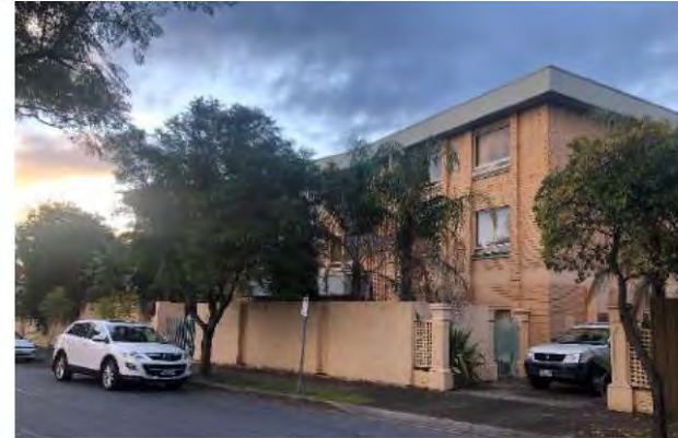
'Elm Tree Lodge' three storey residential flat building looking north-west along Gladstone Street
