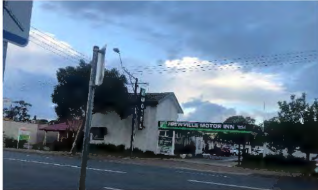
'Frewville Motor Inn' located on the northern side of Glen Osmond Road opposite the subject site.
