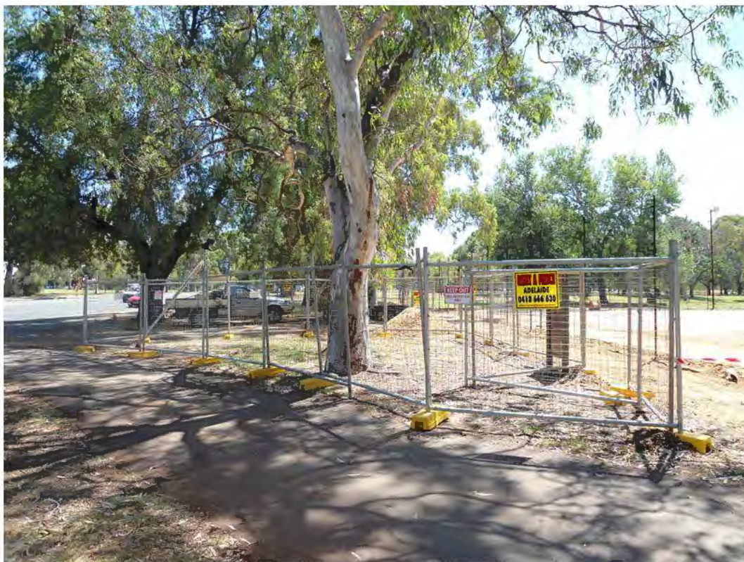
Figure 2: Typical TPZ fencing
