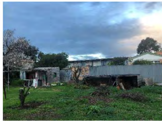
Existing fencing and outbuildings along the eastern boundary adjoining the residential flat building
