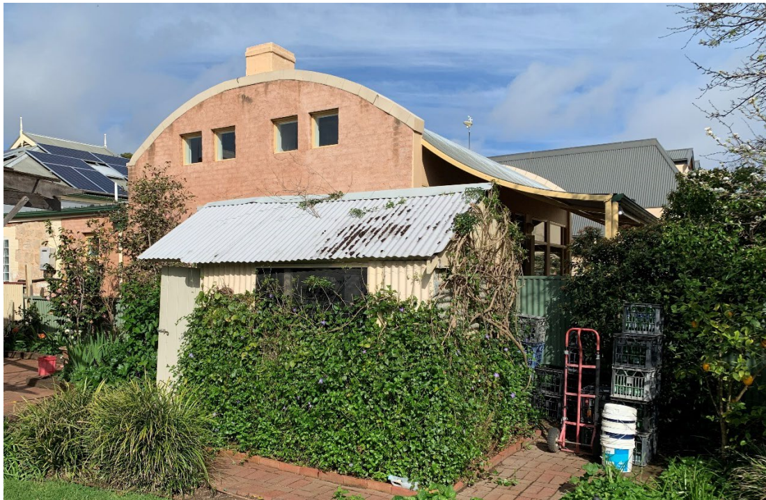
Figure 3: View of the dwelling and verandah at 78 Fairford from the subject site
