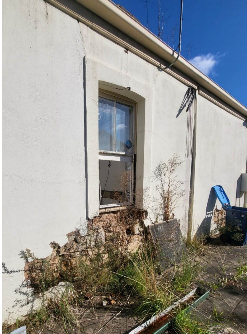
Figure 5: View of the external condition of the dwelling on site.
