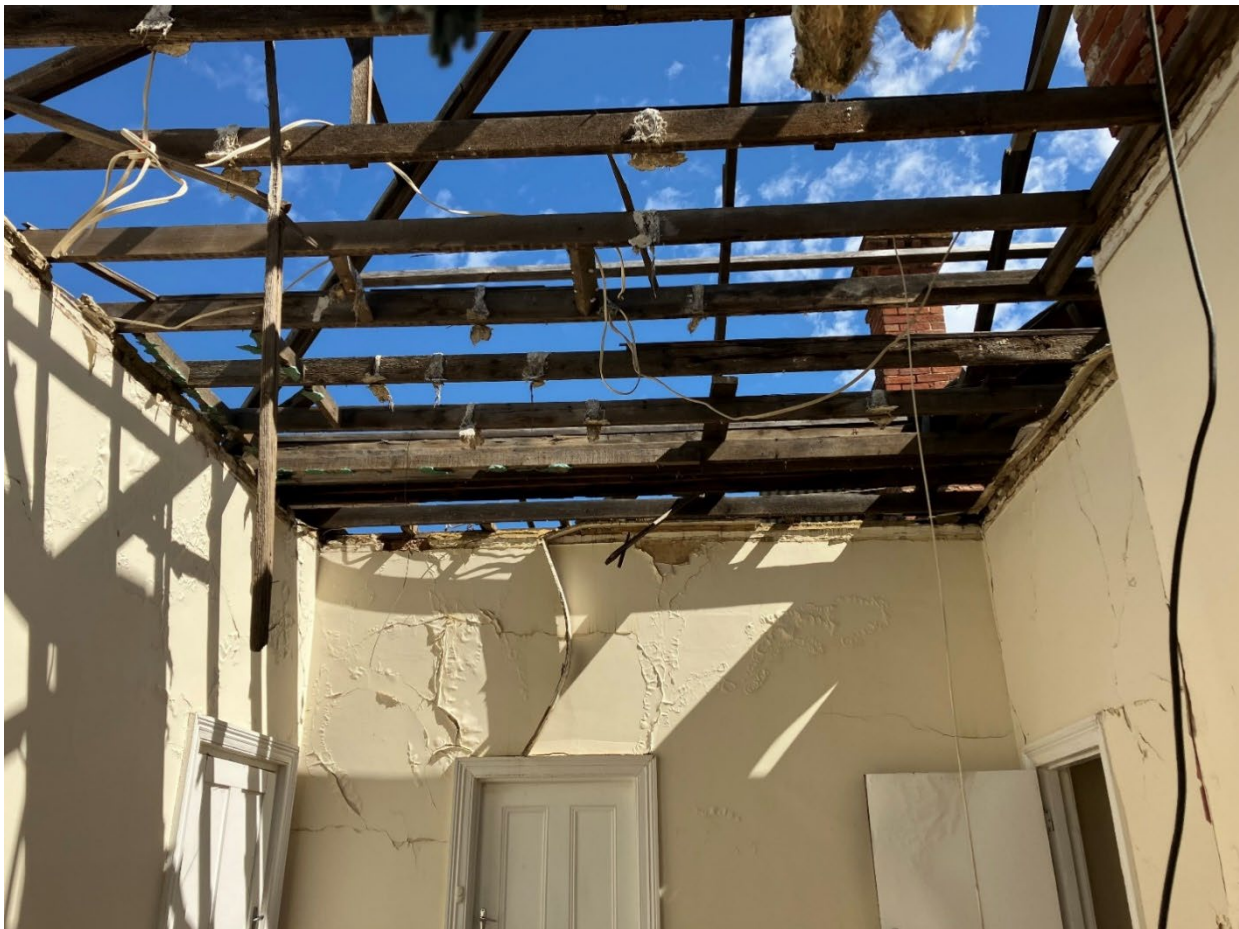
Figure 4: View of the internal condition of the dwelling on site.
