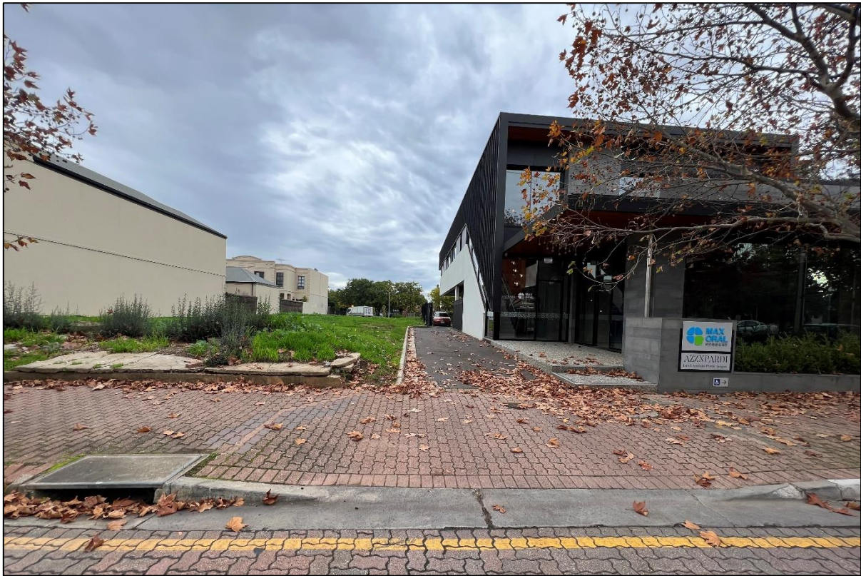
Figure 2: View of the right of way over 4 King William Road as taken from King William Road looking west
