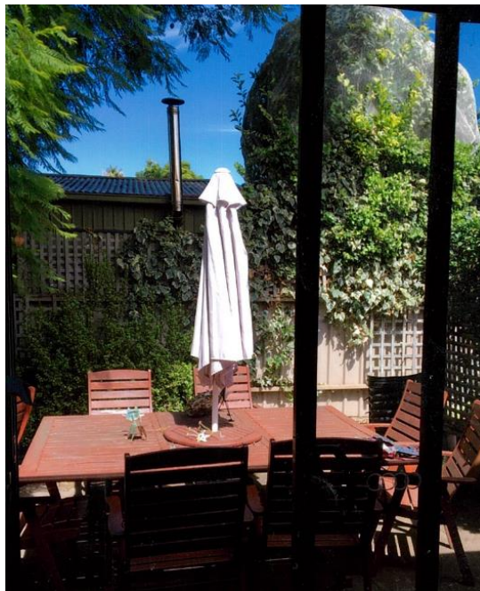
Figure 1: View of the flue from adjoining property when the complaints were received by Council.
