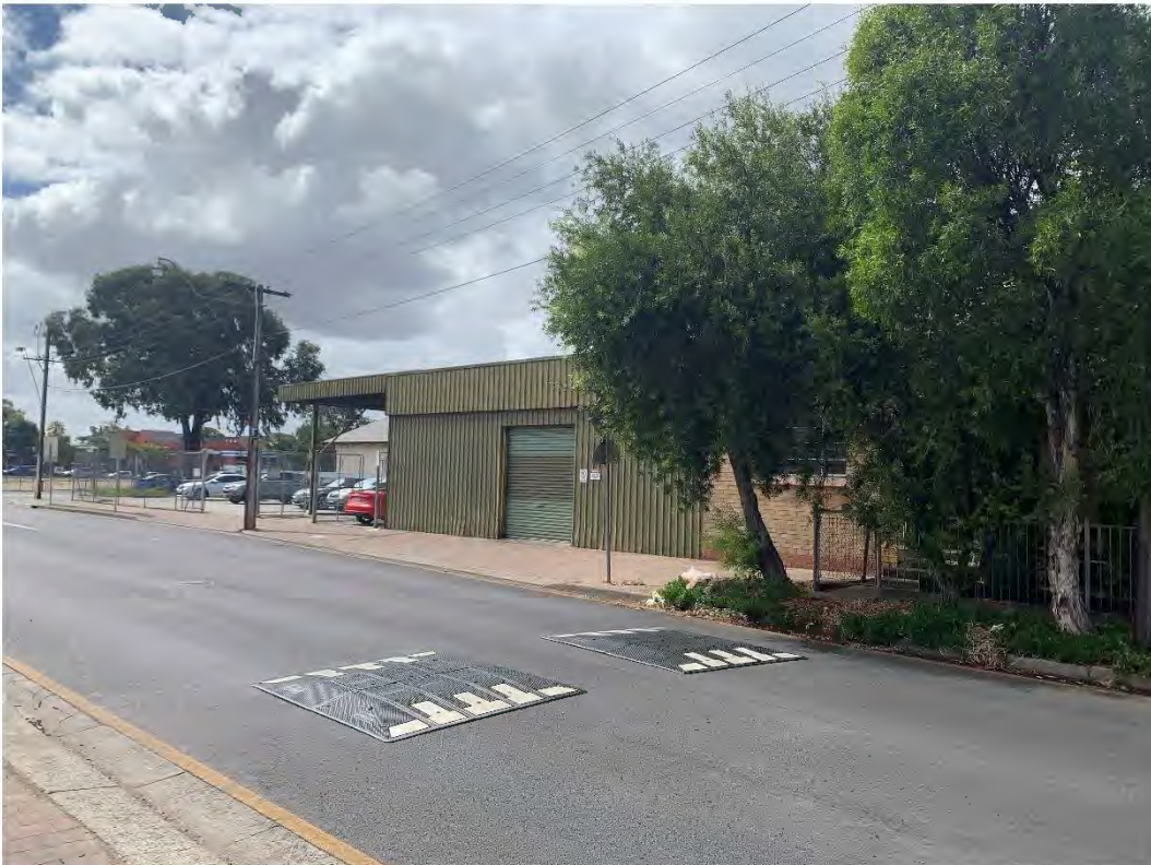
Image 5: Goodman Fielder site on the corner of Leader Street and Leah Street.
