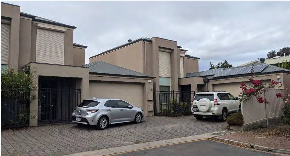
Figure 3: Existing Residential Development at 4-8 Belgrave Court
