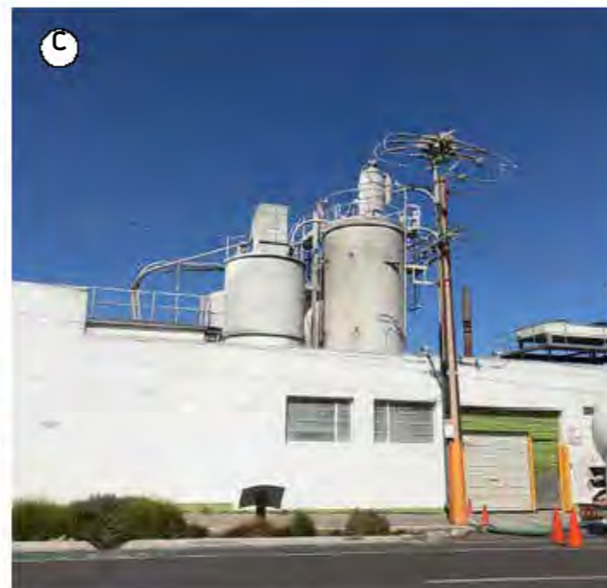
Figure 8: Existing Silos (looking South)
