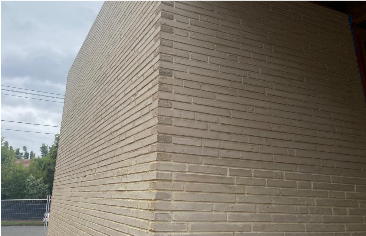
Figure 4 Image of the proposed external materials under construction at a different site.
