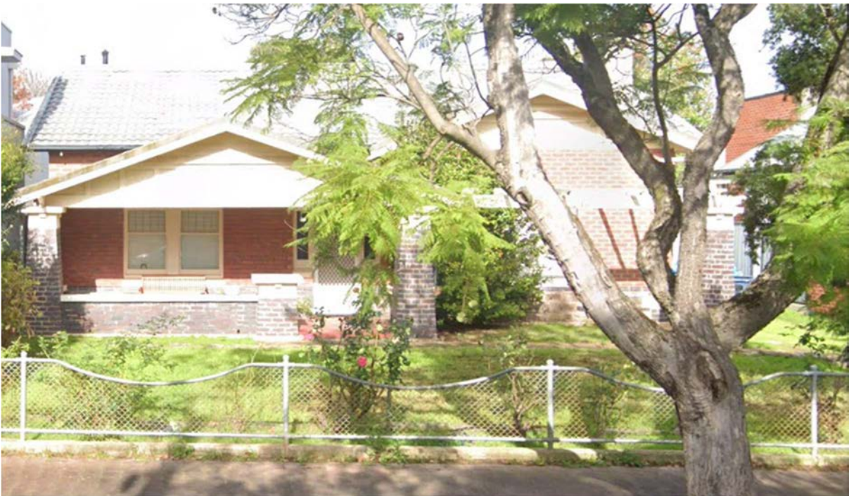
33 Malcolm Street – upper storey in roof space
