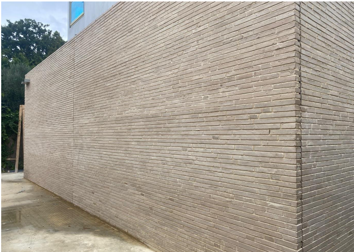
Figure 3 Image of the proposed external materials under construction at a different site.
