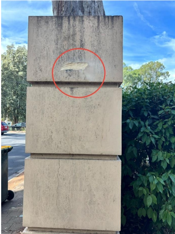
Figures 9 - 10: The gate pillar has been chiselled multiple times to allow gate to shut.
