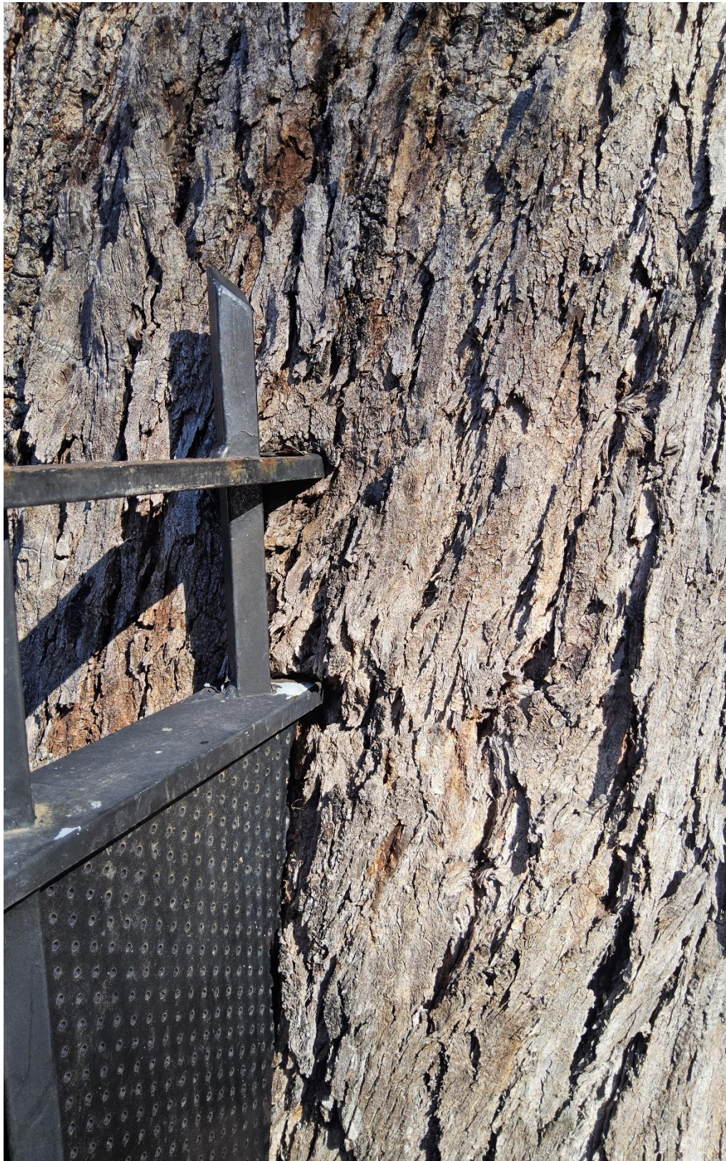
Figure 9. The front fence is embedded into the trunk of the tree and does not show signs of sliding or movement on the trunk.
