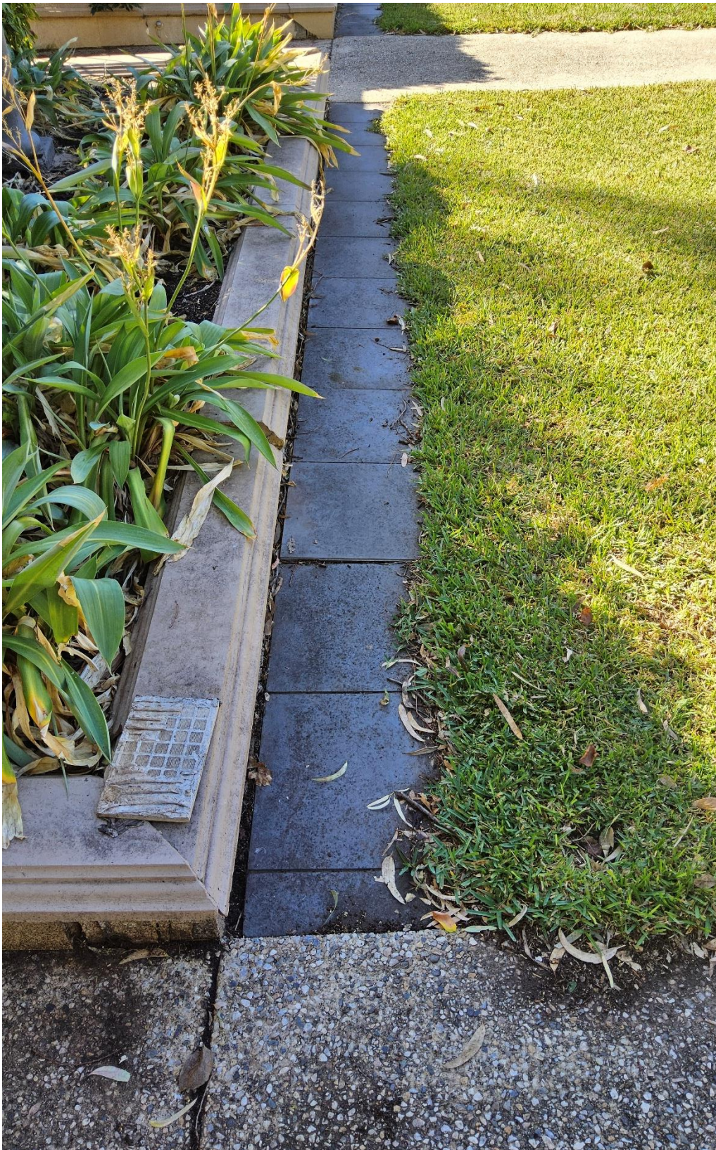
Figure 13. The above shows minor undulation of pavers behind the subject tree.
