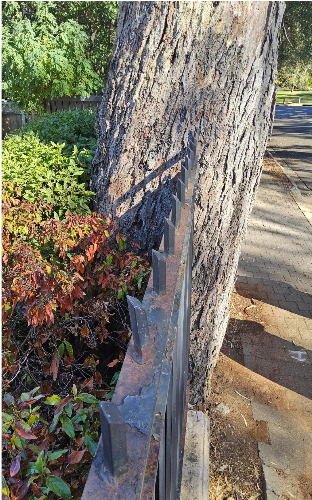
Figure 10. The fence line remains straight with no obvious signs of distortion
