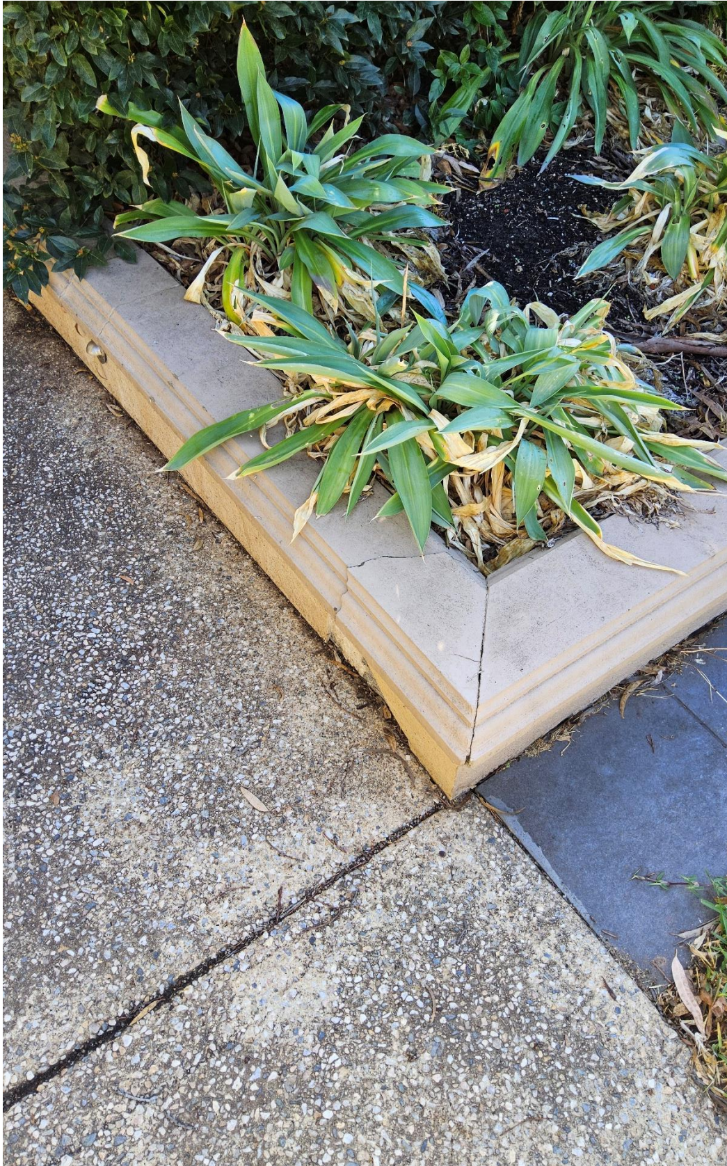
Figure 14. A small hairline crack is noted on a section of the garden retaining wall.
