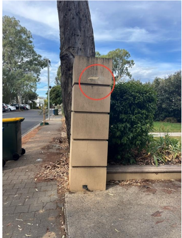
Figures 9 - 10: The gate pillar has been chiselled multiple times to allow gate to shut.
