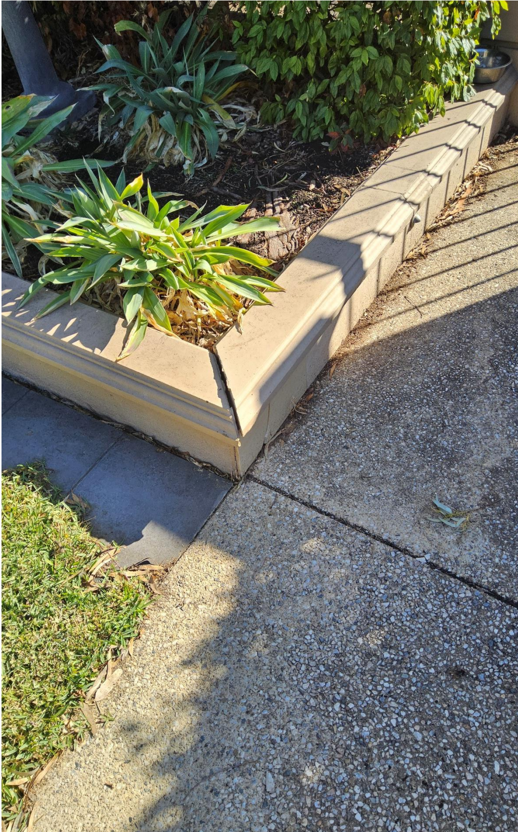
Figure 12. The join between the corner of the retaining wall has separated.
