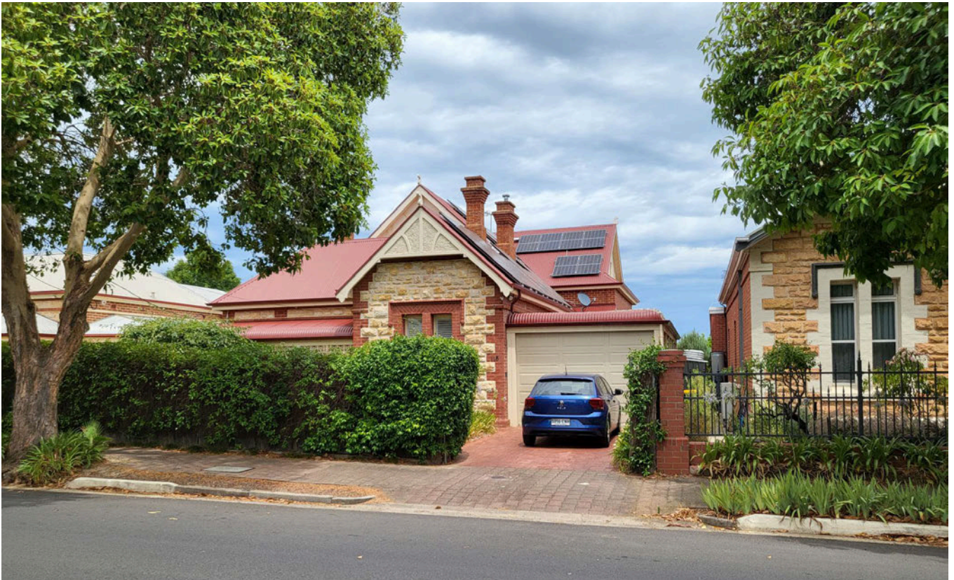
Figure 3: View of the two-storey detached located at 118 Kenilworth Road, south of the subject land.
