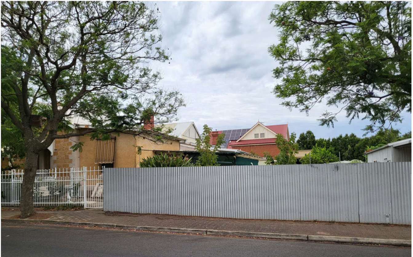
Figure 2: View from the secondary road frontage of the subject land taken from Blyth Street.
