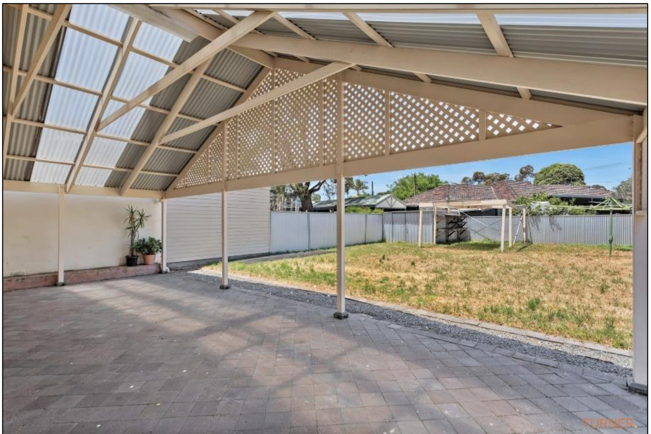
Figures 2 & 3: View of the existing boundary wall of 3 Railway Tce S as viewed from the neighbouring property to the south-west (3 Railway Tce S) – Realeaste.com images
