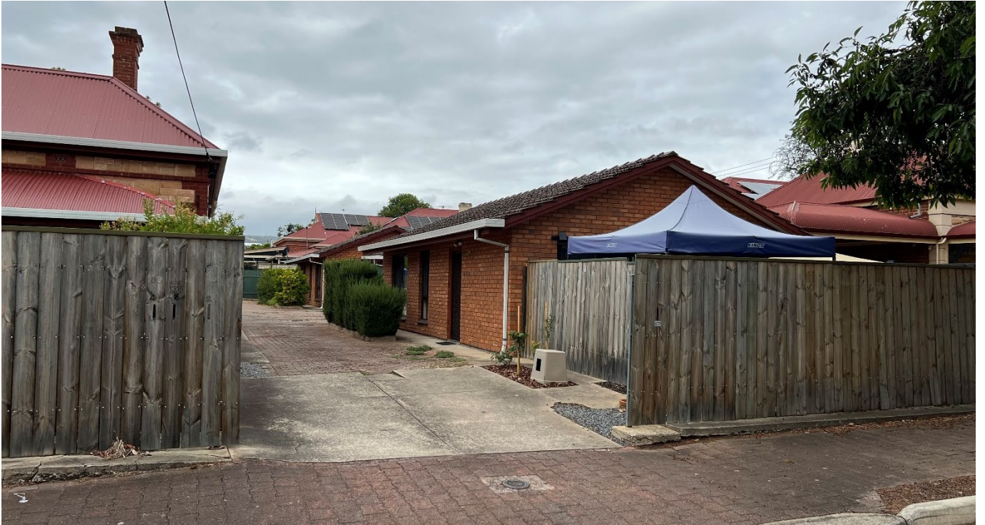
Figure 5: View of the group dwellings at 111 Kenilworth Road, north of the subject land.
