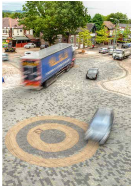
Poynton UK - 'Naked' Intersection and Informal Roundabout. Different pavement treatments indicates roundabouts, street edges and pedestrian crossings.
