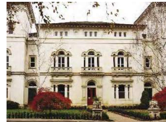
1 Building: Beechworth Lunatic Asylum Location: Beechworth, Vic Function: International Hotel School and accommodation
