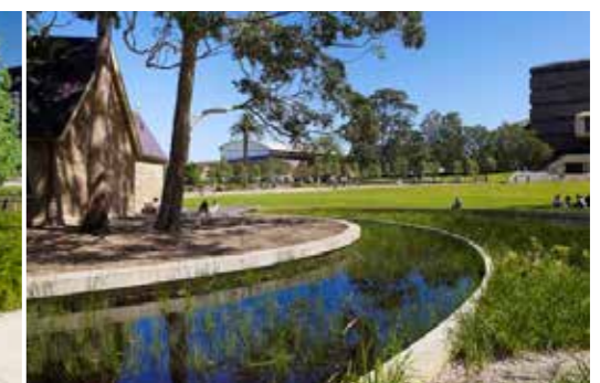
Sydney University, wetland purifies water for reuse in irrigation.
