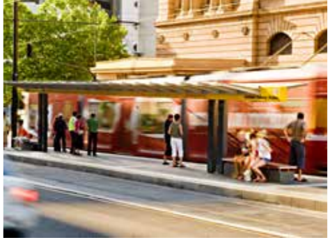
Adelaide Tram Shelters, Adelaide, SA Quality contemporary transport shelters
