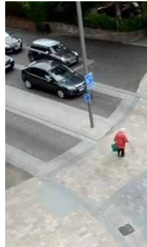
Poynton UK - 'Naked' Intersection and Informal Roundabout. Different pavement treatments indicates roundabouts, street edges and pedestrian crossings.
