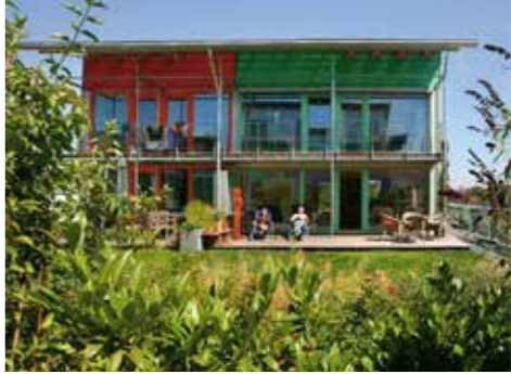
Freiburg Solar City, Germany Communal open 'green' space in mixed use developments
