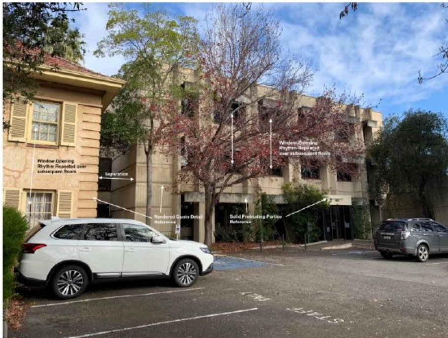
Figure 4, 163A-164 Greenhill Road, Parkside; with notations by Anaglypta Architecture Source: Anaglypta Architecture, August 2022
