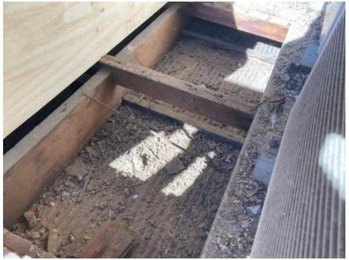
Figure 11 – Northern Balcony Floor Framing
