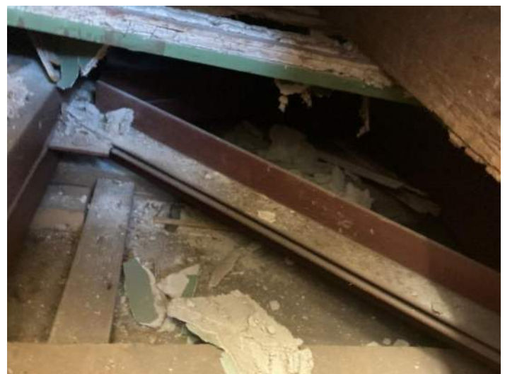
Figure 26 – Steel Bracing Under Western Wing Floor Framing
