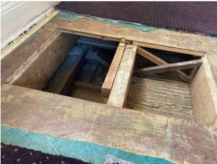
Figure 25 – Western Wing Floor Framing
