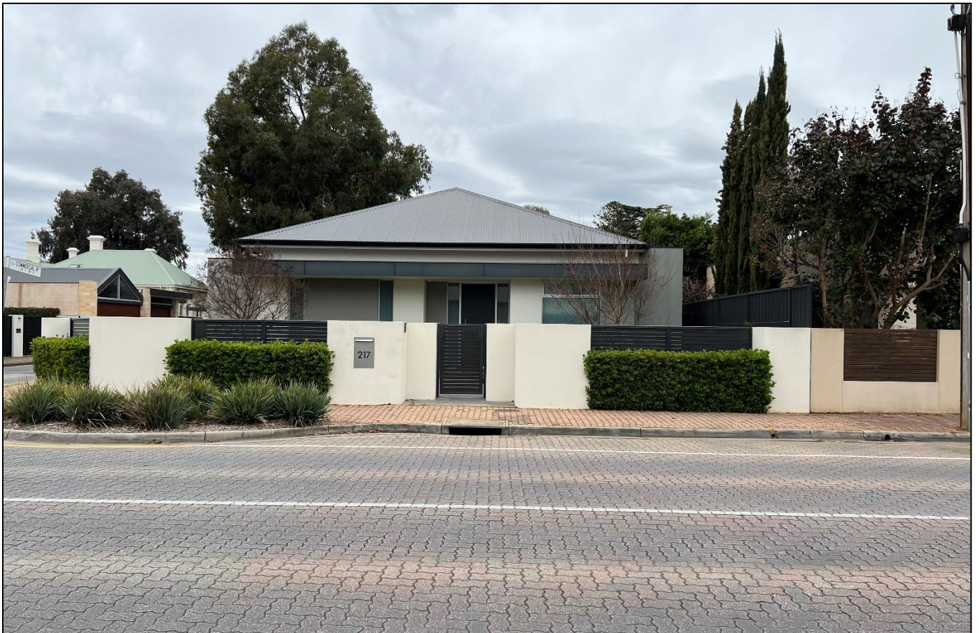
Figure 4: View of 217 King William Road, west of the subject land, as taken from King William Road looking east
