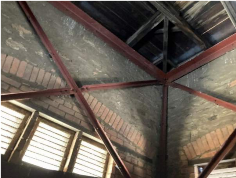
Figure 5 – Strengthening to Central Tower
