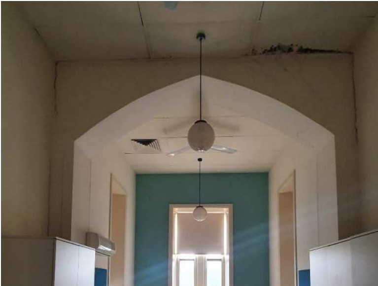
Figure 7 – Central Tower at First Floor Level
