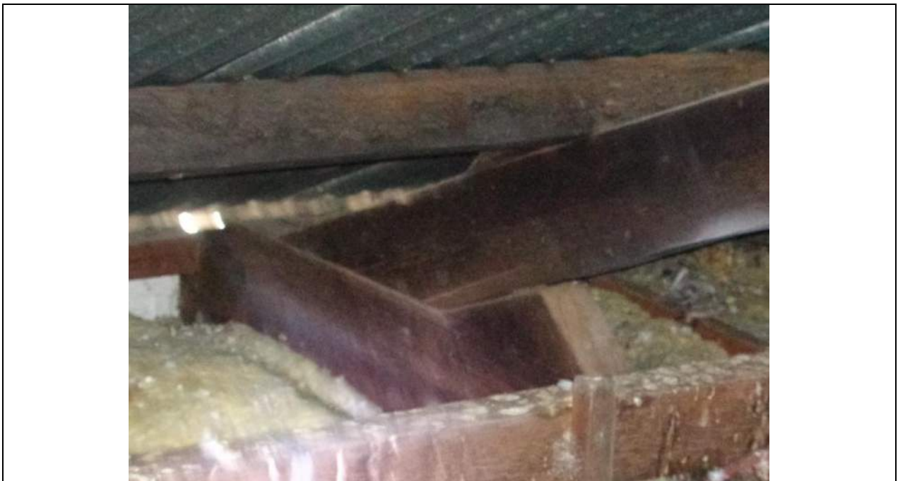
PHOTO 12 – As per photograph 11 above.
