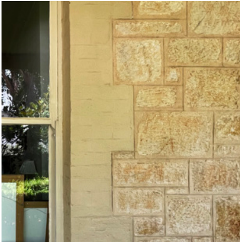
3 -EXISTING TRADITIONAL SAND STONE FACADE WITH PAINTED BRICK DETAILS AND WHITE PAINTED TIMBER FRAMES
