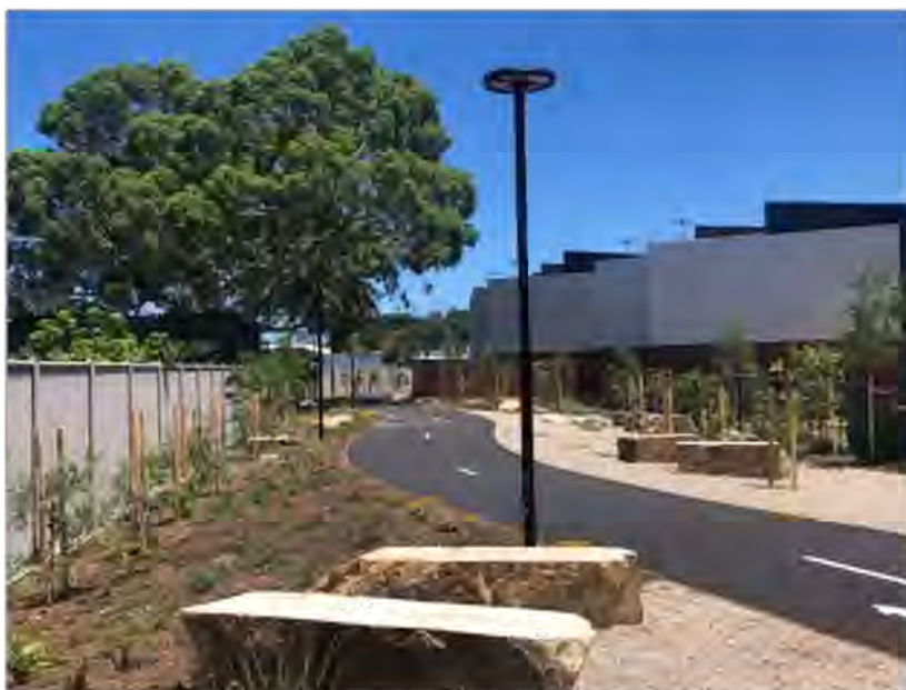
Figure 2.3—Covered culvert at Everard Park
