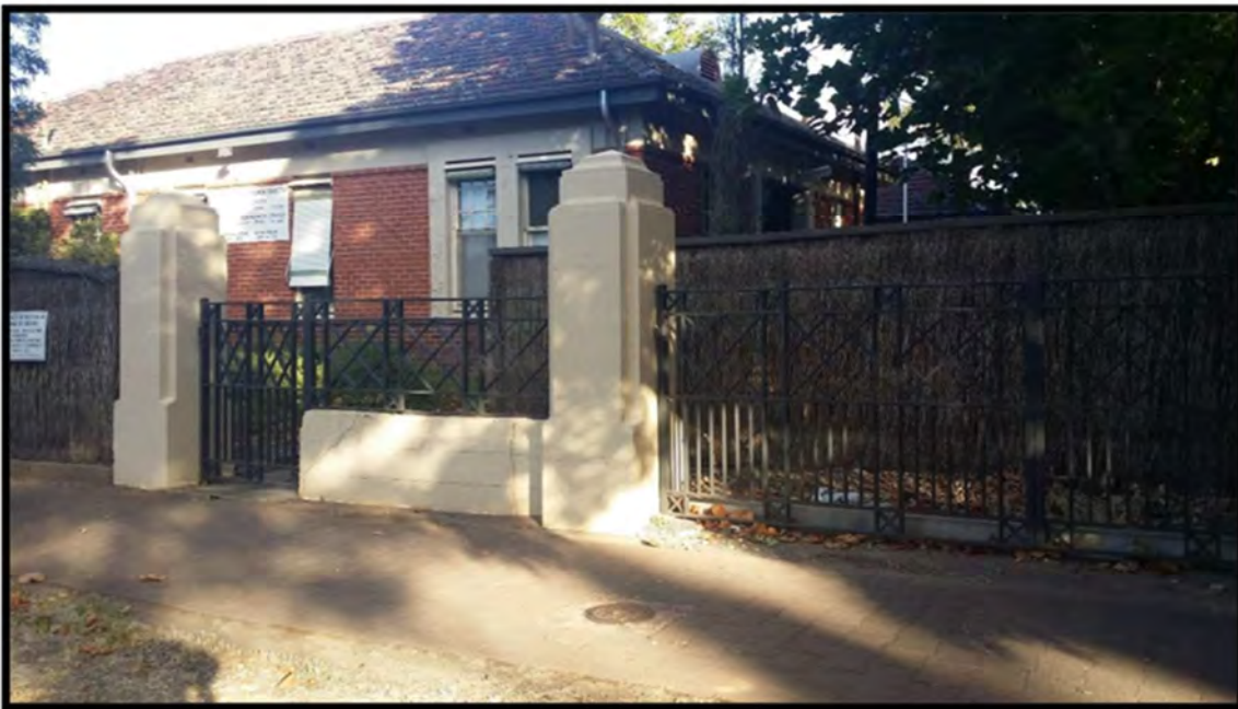
Above: This appears to be a remnant of the original fence.
