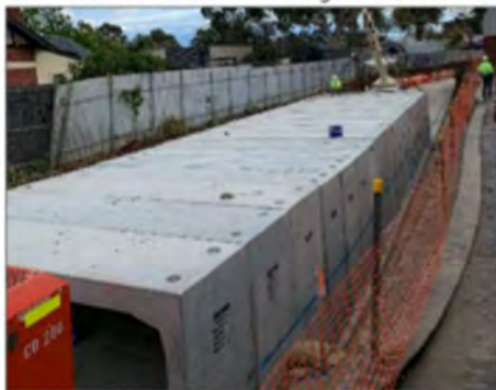
Culvert Installation
