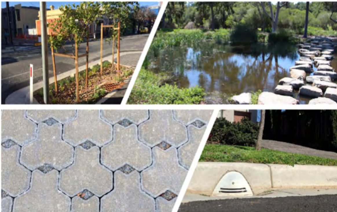
Examples of WSUD in Resilient East – a bioretention system, wetland, permeable paving and a Treenet inlet
