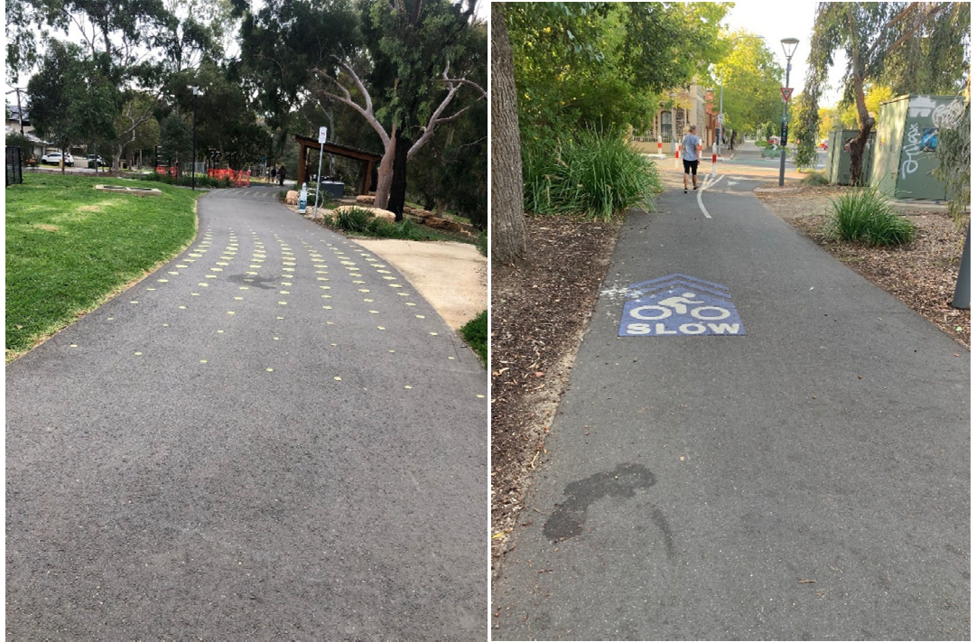
Examples of pavement treatments and decals used on shared paths in Adelaide
