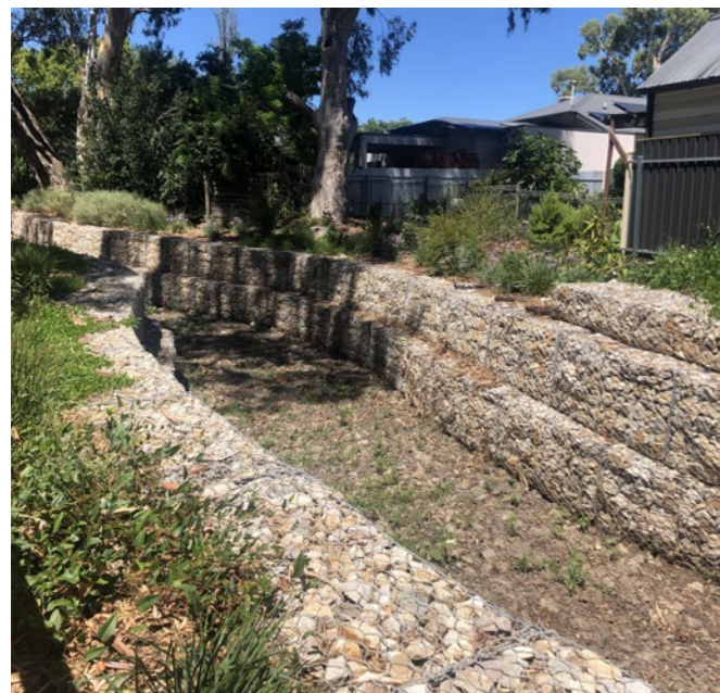
Rock filled gabions
