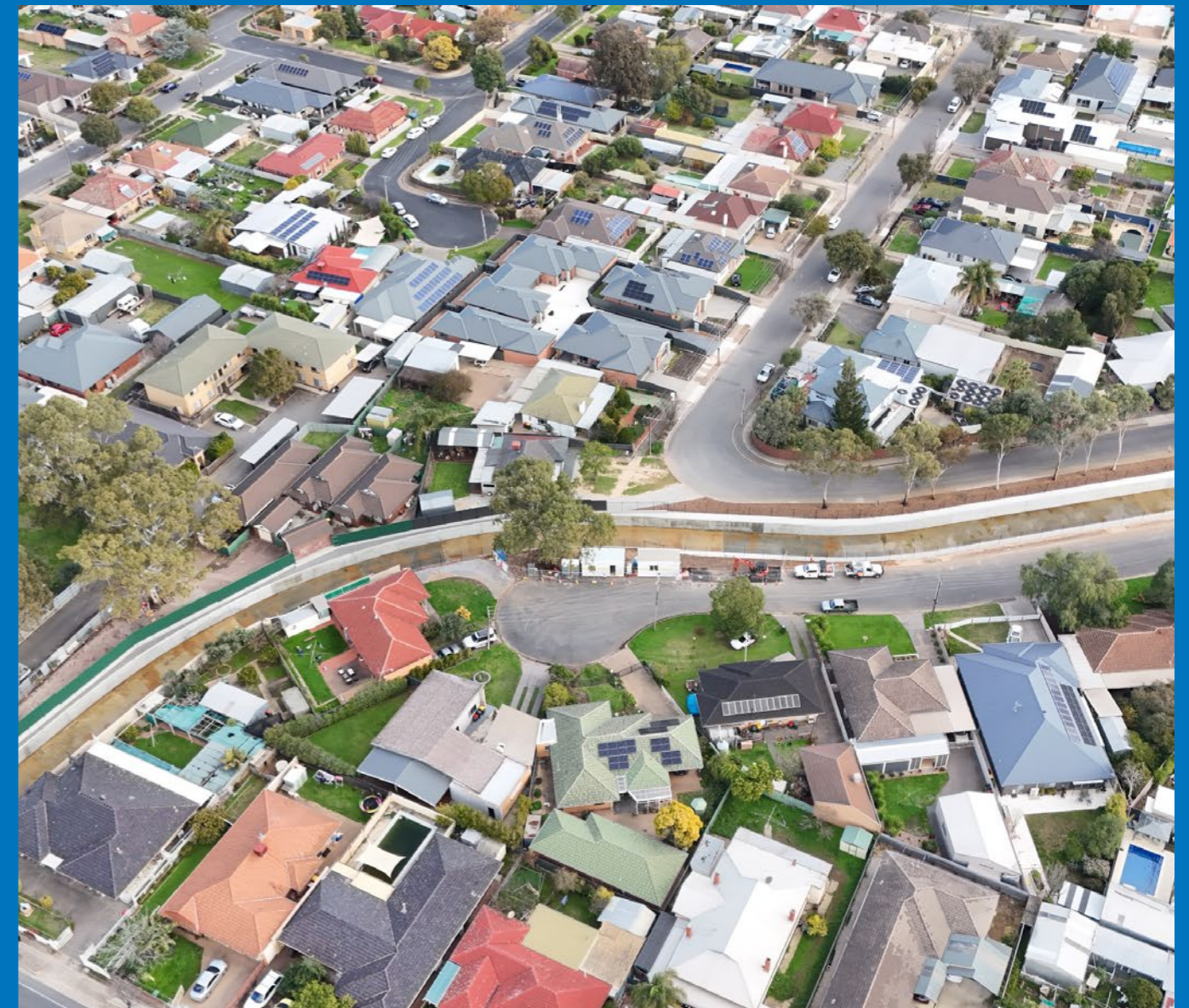
Lower Brown Hill Creek Upgrades
