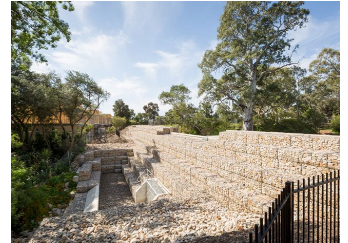
Flood Control Dam
