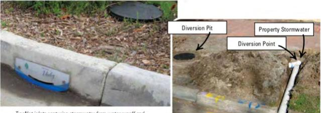
TreeNet inlets capturing stormwater from water runoff and utilise the water to support tree growth.
