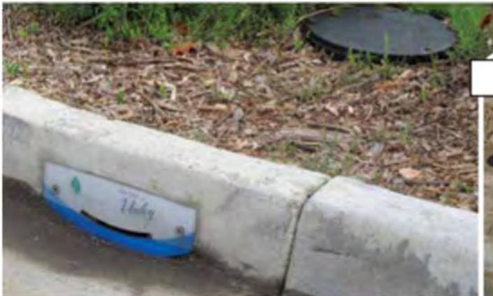
*TreeNet inlets capturing stormwater from water runoff and utilise the water to support tree growth.*
