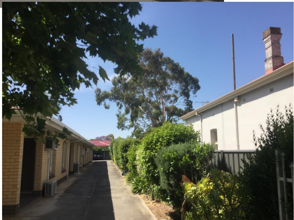
Taken in front of 336 Cross Road, facing north east
