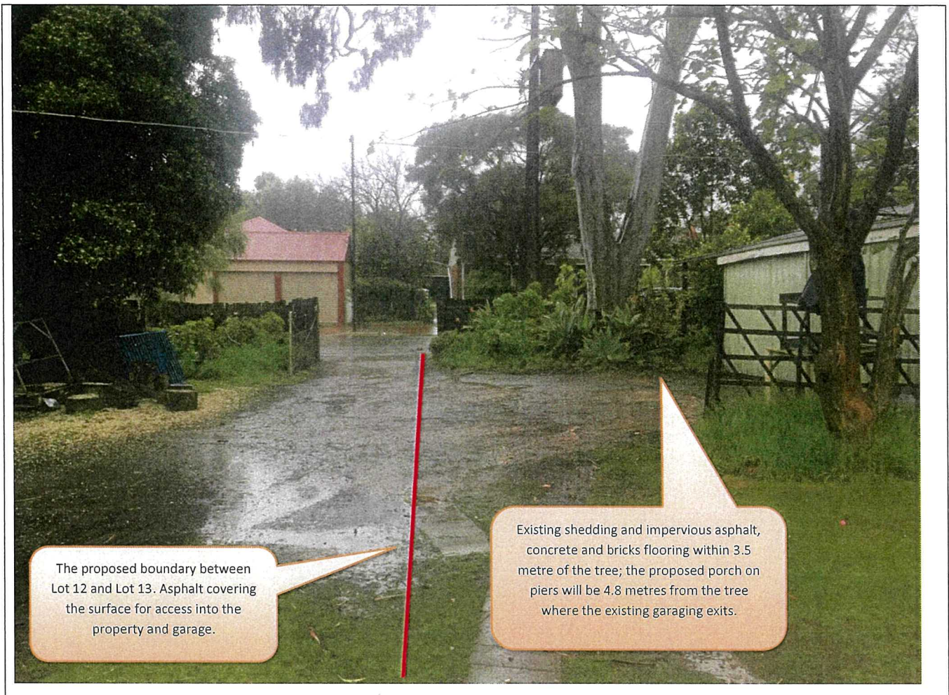
Image 2: The area where the existing shedding and garaging will be removed to a depth approximately 50-100mm depending on the concrete, pavers and or asphalt without damaging tree roots or adversely affecting the health of the tree. Consequently it is unlikely that tree roots will be located in the area identified for footings as depicted on the indicative dwelling plans.
