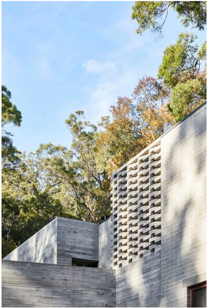
MW-P PERFORATED MASONRY WALL FACE BRICKWORK
