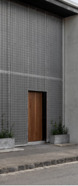
MS METAL SCREEN TO UPPER LEVEL WINDOW. WEBFORGE GRATE OR SIMILAR THE SCREEN FILTERS LIGHT AND PROVIDES PRIVACY
