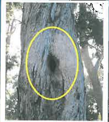
Trunk degradation and breach. Note the minor trunk swelling at the area of structural inadequacy.
